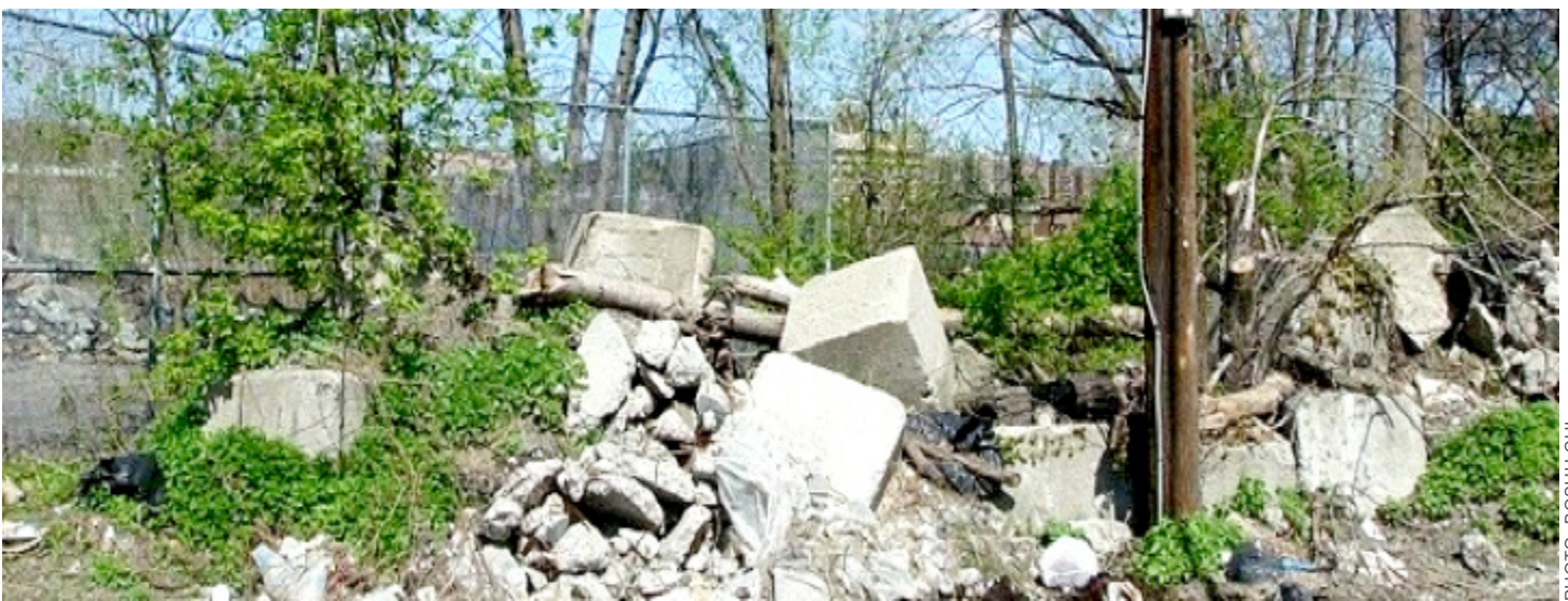
Above: Photograph of debris along Exterior road spanning the DCAS and Con Ed sites.
