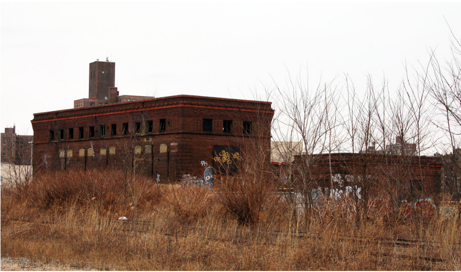
Left: Abandoned historic transformer house on the MTA property (1907).
