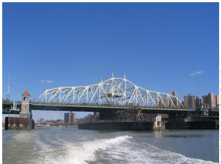
Below: The University Heights Bridge
