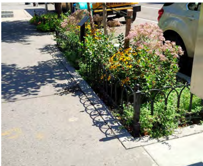
Street bio-swales installed by DEP and NYC Parks could help reduce combined sewer overflows in certain drainage areas outletting to the Harlem River
