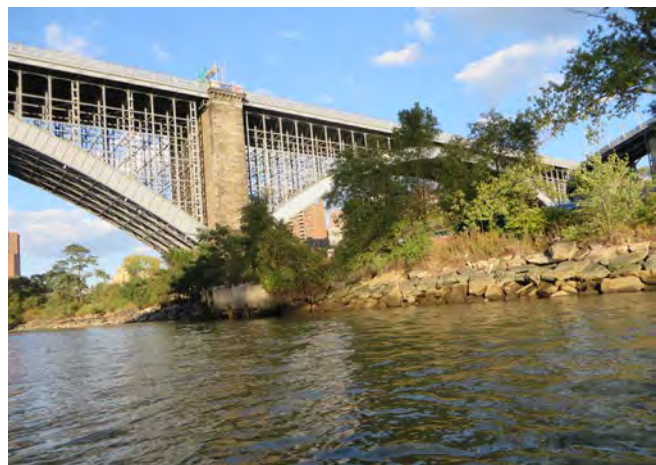
The Bridge Park segment of the Harlem River Greenway offers shoreline habitat while protecting the shoreline from erosion with riprap; bike path is beyond
