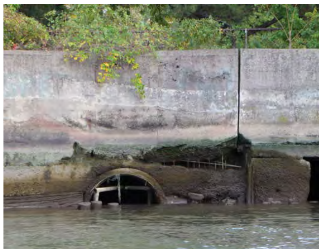
Combined Sewer Overflow near RCSP
