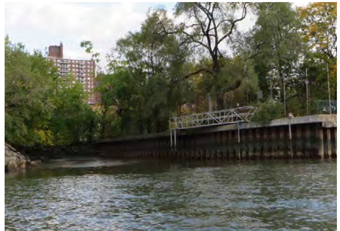
Bulkhead at RCSP damaged by Superstorm Sandy before reconstruction and replacement of some portions with a more naturalized shoreline
